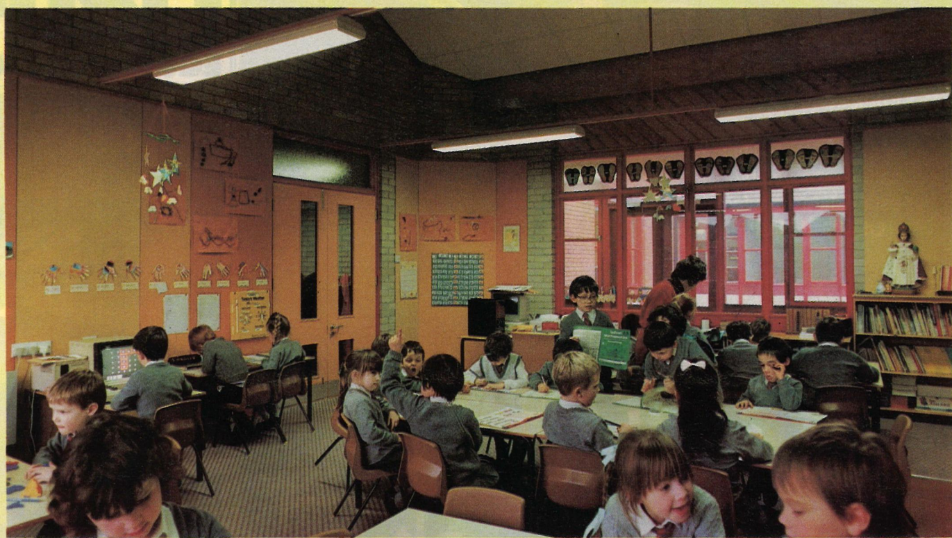
The recently built St Dominic's Primary School in Stone, Staffordshire has been equipped with Sylvania Syl-Louvre white aluminium reflector fluorescent fittings. These fittings were specified to provide a lighting level throughout the classrooms and corridors of between 350-500 lux, while avoiding glare, as all classes make extensive use of computer screens.
